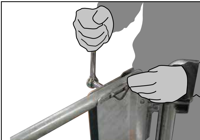
I. Once the gate is lined and levelled tighten the hex nuts and bolts on the top & bottom guardrails using a 3/16" Allen Key and 1/2" socket.
