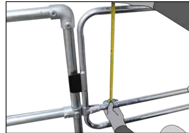
Q. Use a measuring tape to ensure gap between top rail and mid rail is no more than 470mm. Adjust if necessary.
