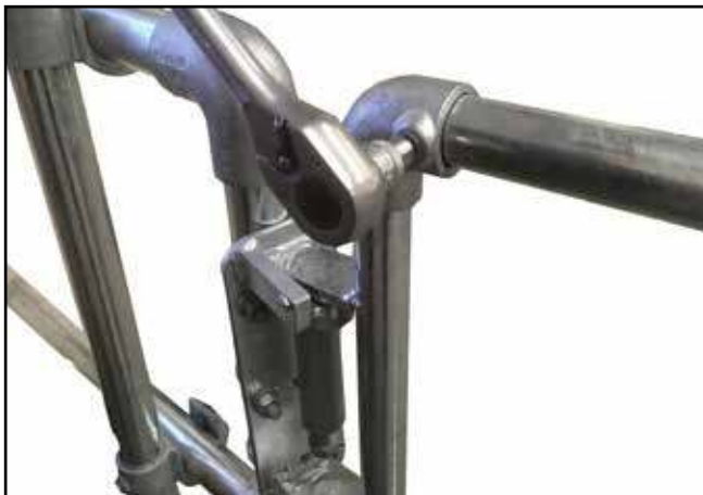
G. On left hand gate disconnect the tubular gate from the hinge assembly by loosening the top & bottom cast clamp grub screw using a hex head socket as shown. This and the following 3 steps will also be repeated for the right hand gate.
